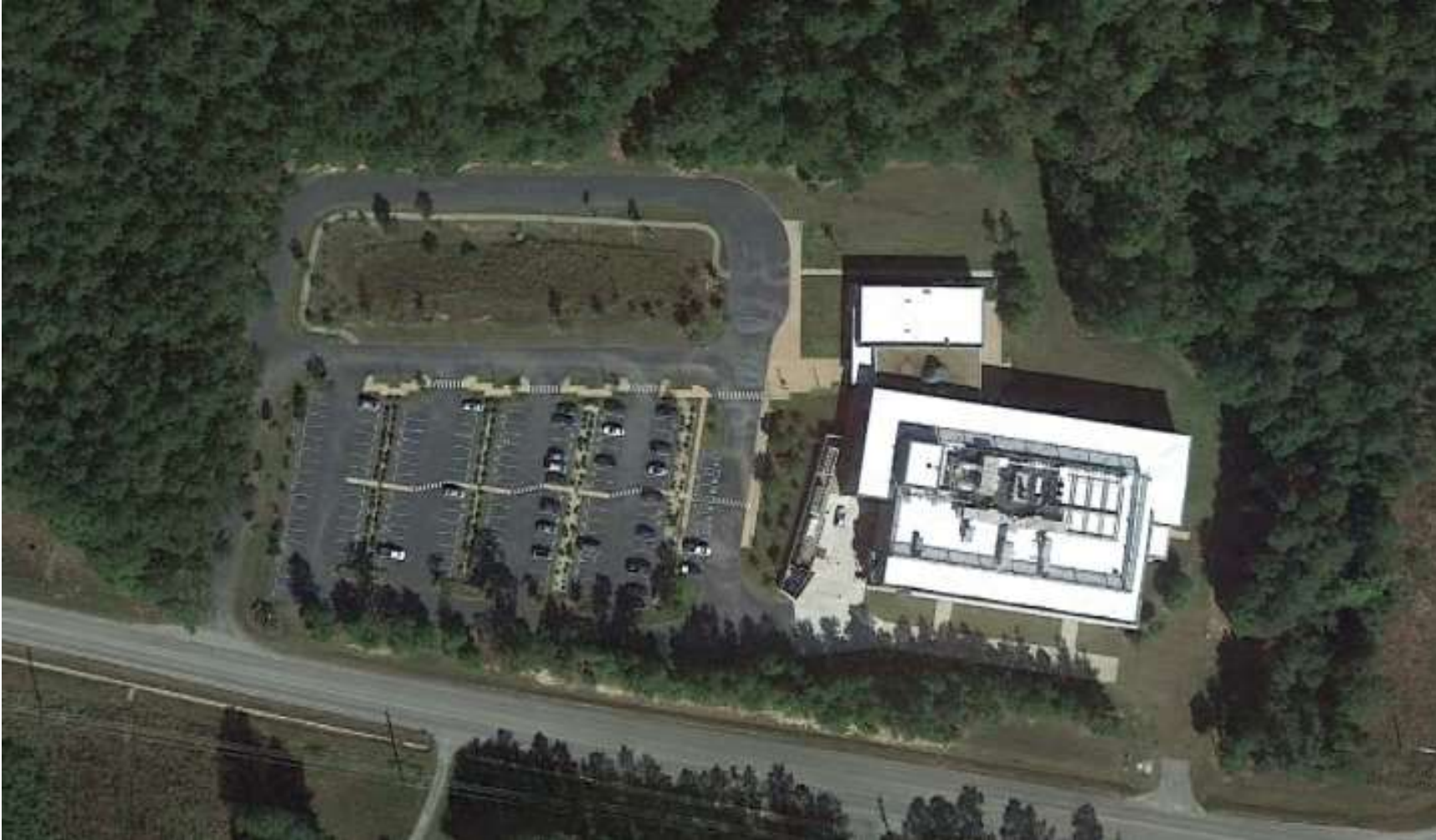
Commonwealth Center for Advanced Manufacturing 10+/- acre site
