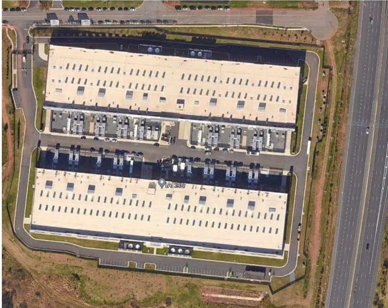
Generic Commercial Data Center (Loudoun County, VA) 22+/- acre site
